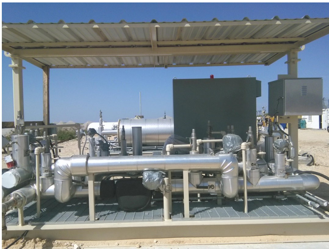
Figure 6. Pump skid.
