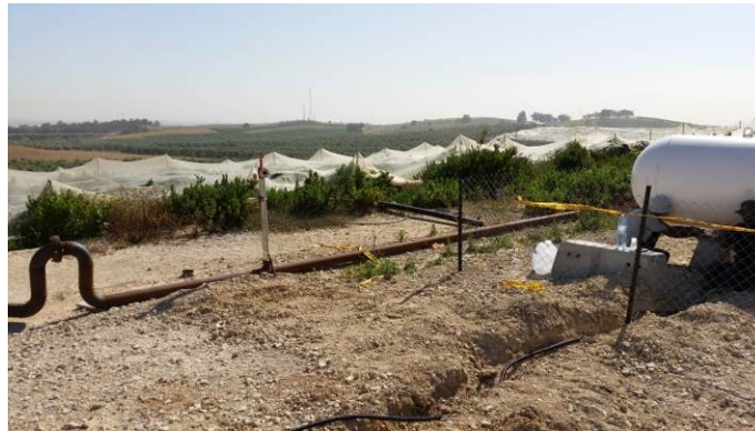
Figure 15. For fire safety reasons, a water pipe line surrounds the site. Two hydrants are installed on the pipe and near them a fire cabinet (cannot be seen in the image).
